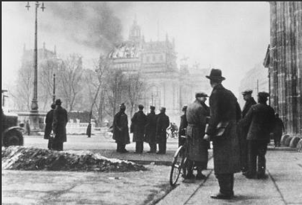
Onlookers in front of the Reichstag (German parliament) building the day after it was damaged by fire. Photo credit: USHMM and Bildarchiv Preussischer Kulturbesitz.
